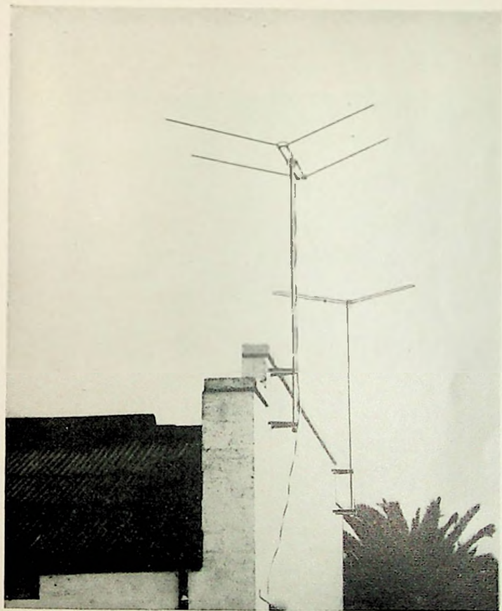
Plate VI. Double V and folded V aerials for multi-channel reception of horizontal polarization
