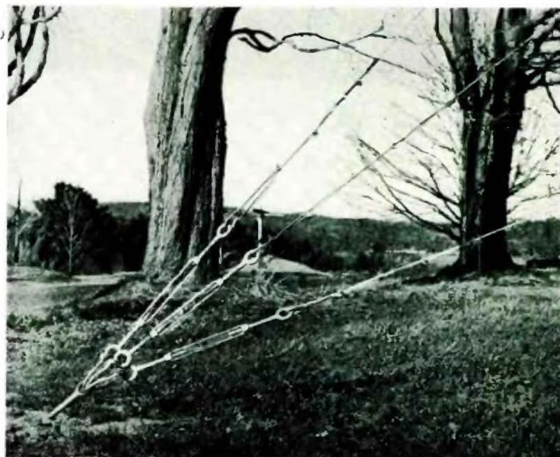
Fig. 15. The final arrangement of the guy wires and turnbuckles
