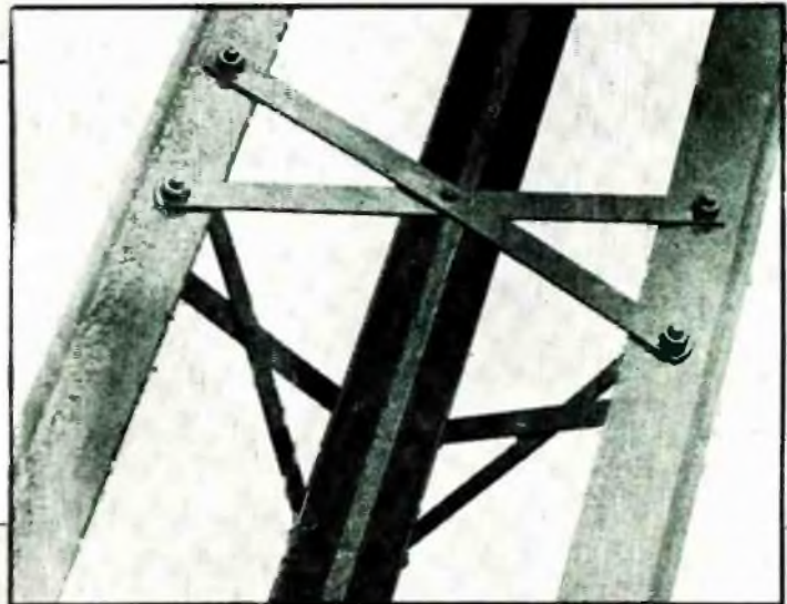
Fig. 6, below. This section carries three saddles to which the guy wires will be fastened
