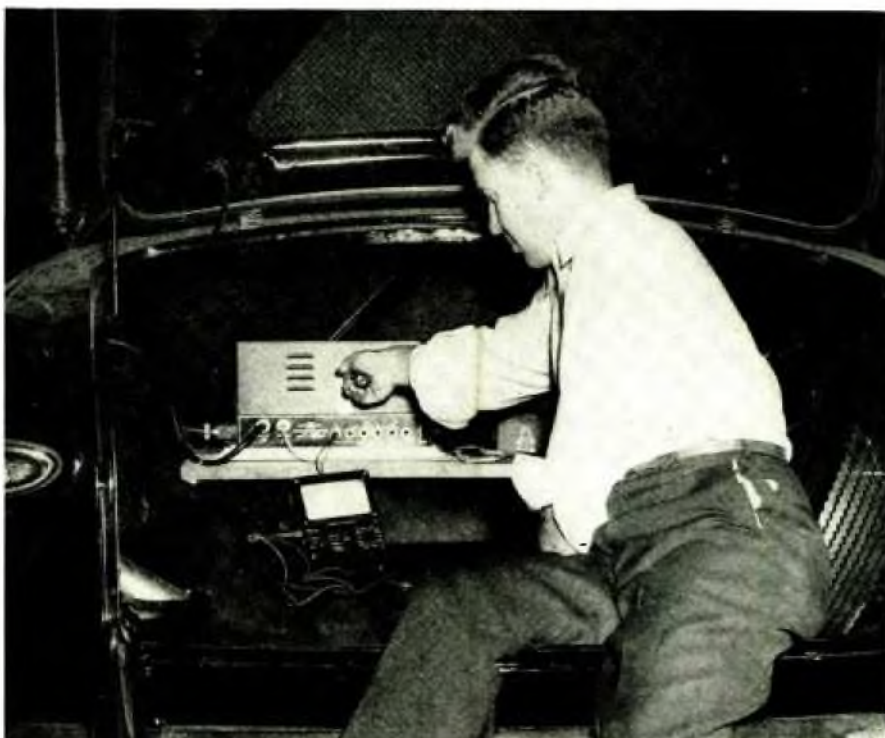
Fig. 6. Equipment is mounted above rear compartment deck as protection from water
