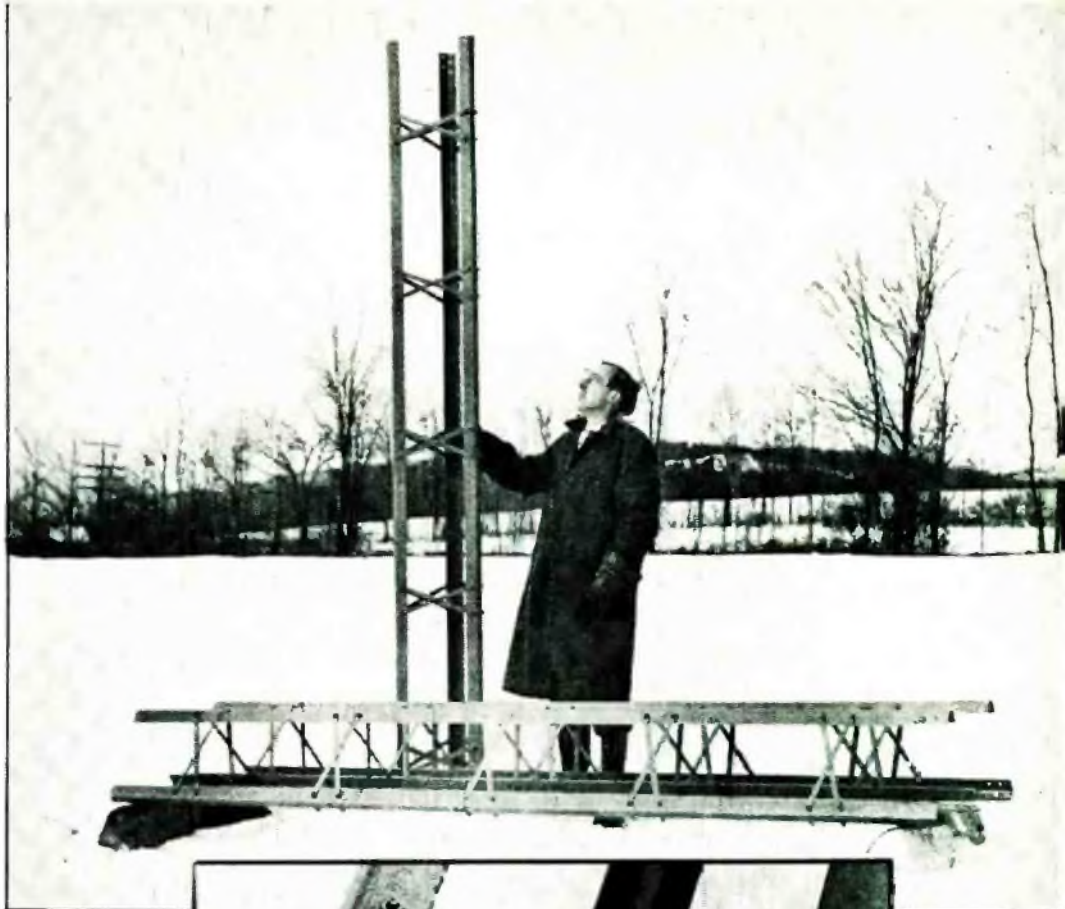
Fig. 4. Two assembled sections of the tower, ready for the first coat of paint
