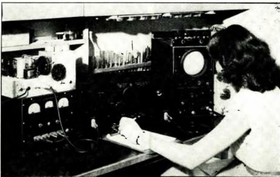
Fig. 25. Browning calibrator setup for the test position of an assembly line
