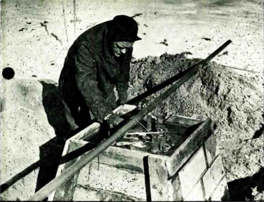
Fig. 10. The base plate levelled and trussed up in the fresh concrete
