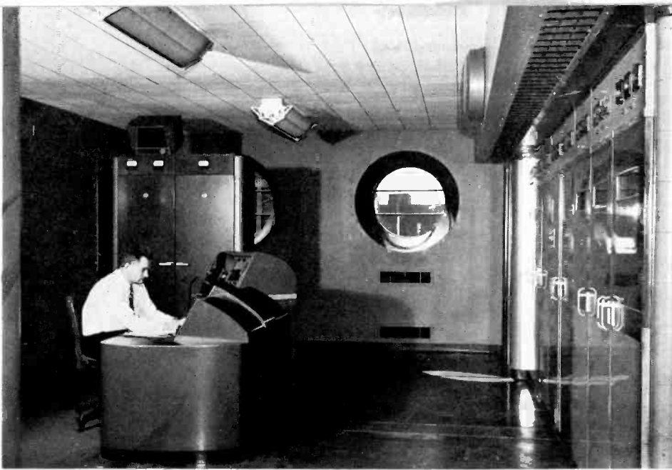
The supervisory control console, equipment racks and flush mounted RCA transmitter in St. Louis' KSD-TV transmitter room (plan shown above right). Key to the floor plan of the transmitter room is: A & C—equipment racks, B—TV console, E—tube rack, F—diplexer and dummy load, G—sideband filter, H—TV transmitter, J—water circulation pump. At right is the transmitter room of WHIO-TV in Dayton, Ohio.
