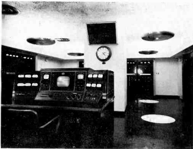
(Above) Some of Dumont Television Network's new transmitter equipment on the 82nd floor of the Empire State Building showing the main control console. In the background to the left is the regular transmitter, the spare transmitter is at the right. (Right) A section of the utility area at WHIO-TV in Dayton, Ohio.
