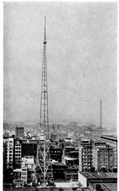
An antenna tower located as this one is in a city must usually be self supporting. Self supporting towers are more costly than the guyed type, but usually permit easier inspection and maintenance.
