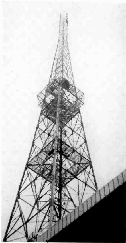
The 550-foot self-supporting tower of JOAX-TV, Tokyo, is attached directly to the studio building and contains an elevator to the 280-foot level.
