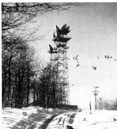
Fig. 1-27. Microwave relay station at Green Pond, N.J.
