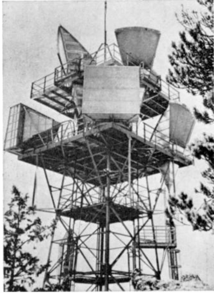
FIG. 1-26. A radio relay tower used for the reception and transmission of television signals.
