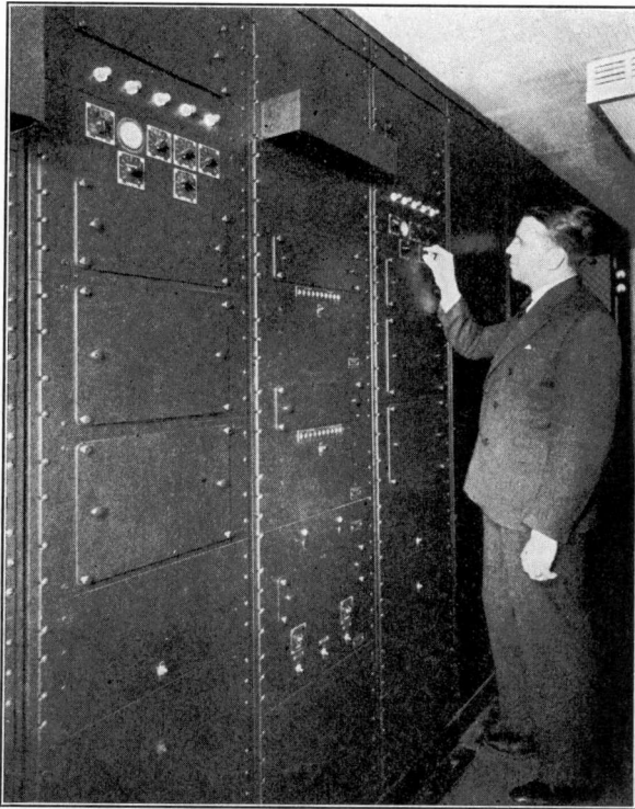
FIG. 18.12.—Synchronizing Generator and Video Line Amplifier Panels (courtesy of NBC).
