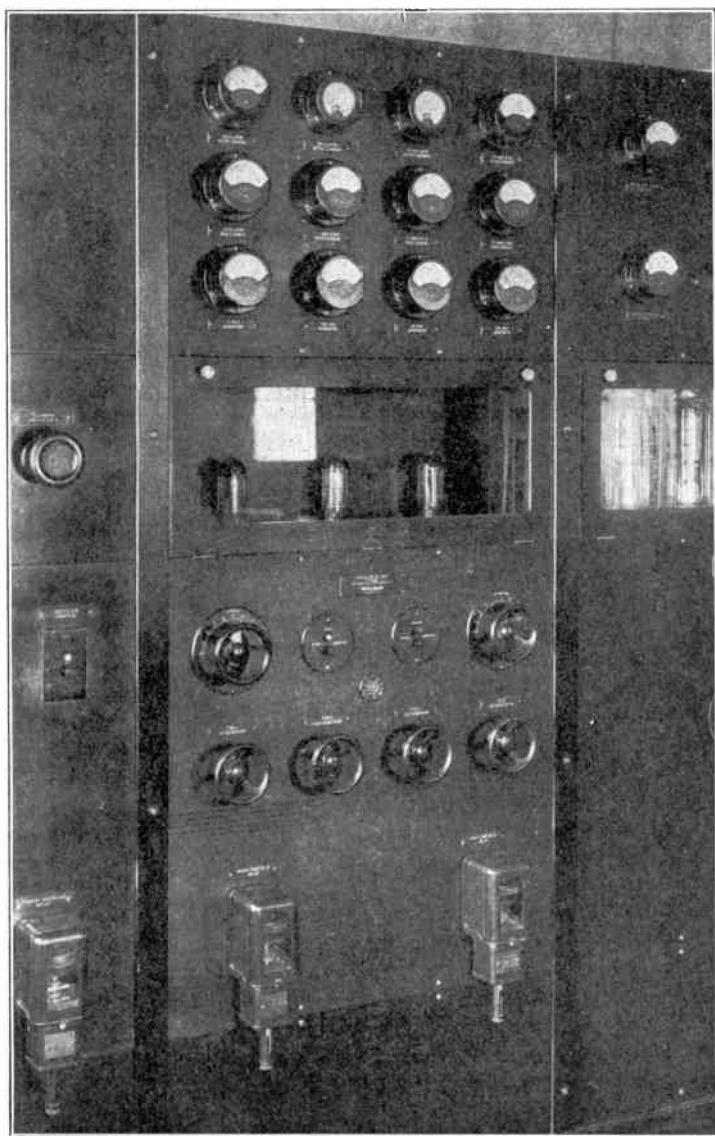
FIG. 222. Master Oscillator Frequency Stabilizer Panel.
