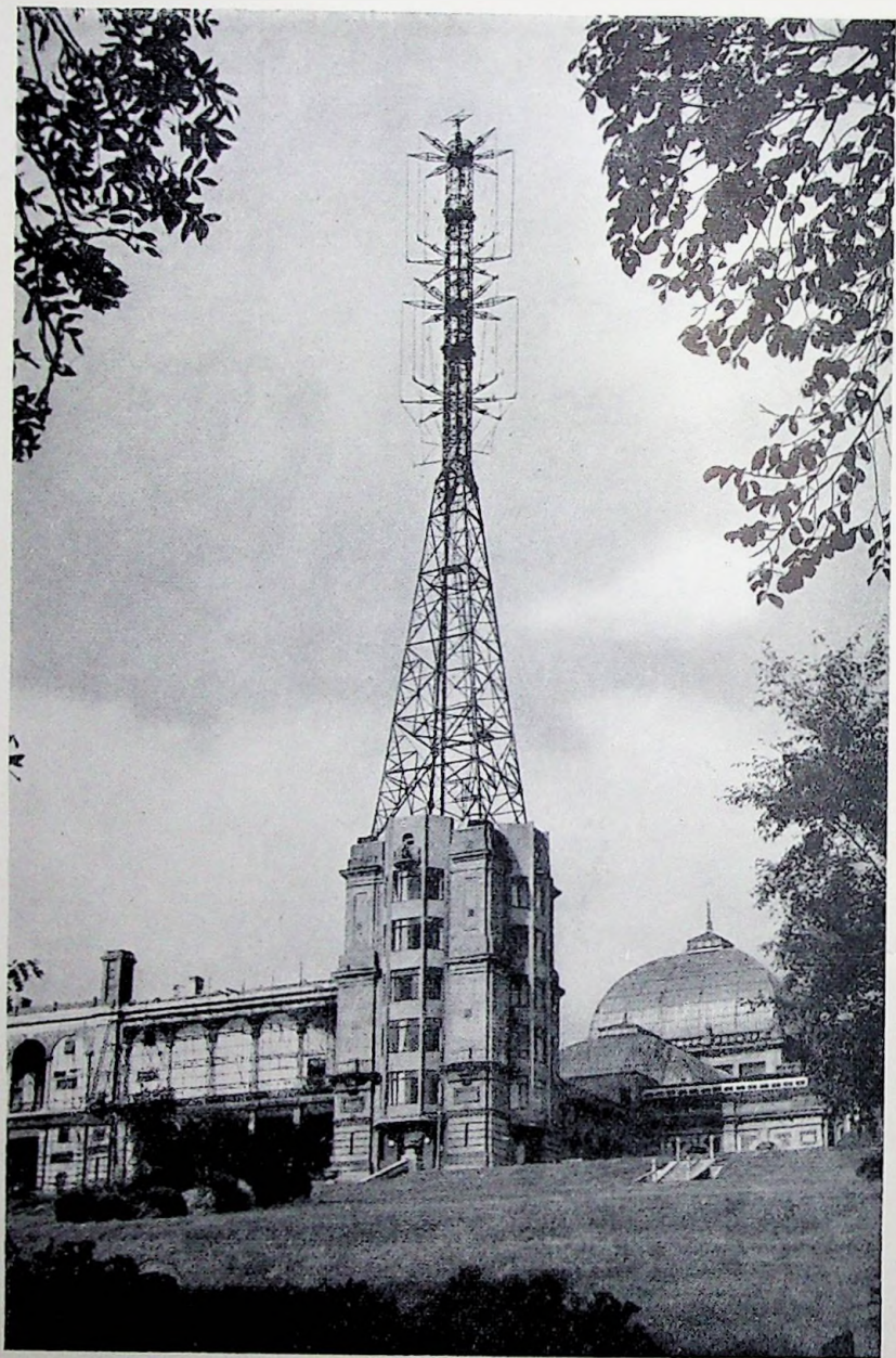
Frontispiece: THE AERIAL TOWER OF THE B.B.C. TELEVISION TRANSMITTER AT ALEXANDRA PALACE, NORTH LONDON (Courtesy of the B.B.C.)
