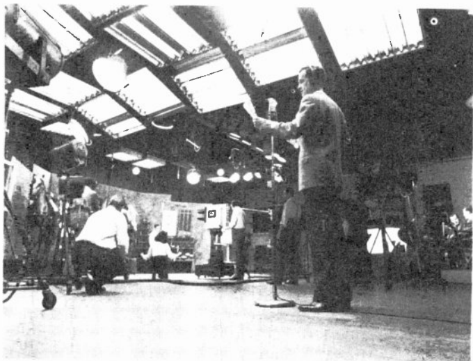
Figure 8. A studio equipped with fluorescent lighting. (courtesy CBS)
