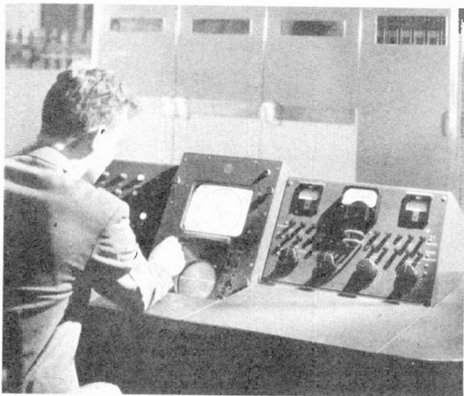
Figure 128 Monitor facilities for checking video transmitter. (courtesy RCA)
