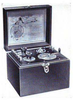
A simple vacuum tube receiver which operates from a single dry cell
