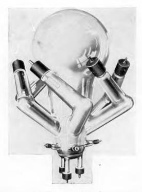
Fig. 69.—A.E.G. HEXAPHASE GLASS BULB RECTIFIER.
