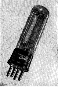
FIG. 1-5. A typical phototube.
