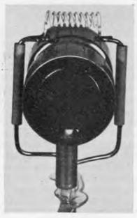
Fig. 67.—Directly Heated Spiral Cathode of a Low-voltage Rectifier. (Current density 3 amp./cm.²; AEG N 190/10; \(\frac{3}{4}\) natural size.)
