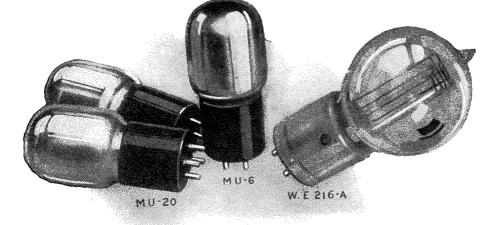
The MU-20 tubes shown above are designed specifically for use in resistance- or impedancecoupled A.F. amplifiers. They have an exceptionally high amplification factor and a high output impedance. Both the MU-6 and the W.E. 216-A are power amplifiers for use in the last stage of any type of A.F. amplifier They both have a low output impedance.
