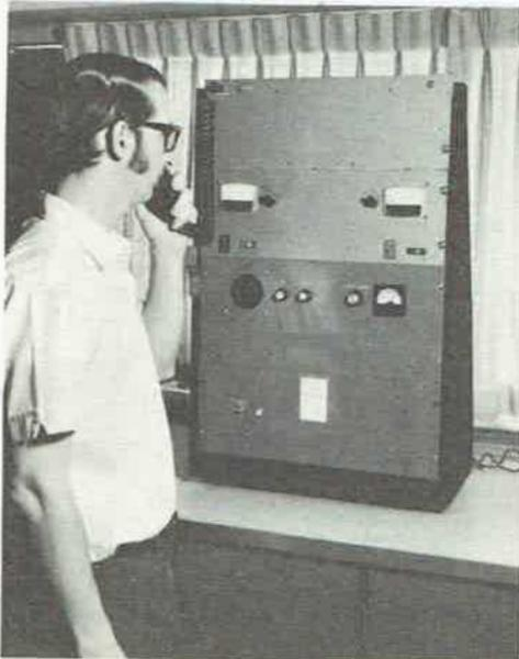
Fig. 12-4 - W1FBY tries local control on a 450-MHz repeater. This "machine" uses transmitter and receiver decks from the Motorola T-44 series mobile transceivers.
