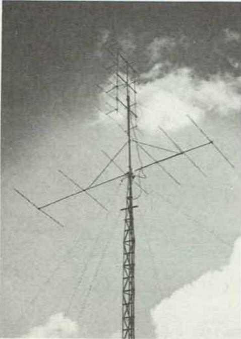
Fig. 9-12 — A 6-element Yagi for 50 MHz, with optimum spacing for forward gain given in Fig. 9-13. Boom is 20 feet long. Antenna at the top is 16-element all-metal collinear array for 144 MHz.
