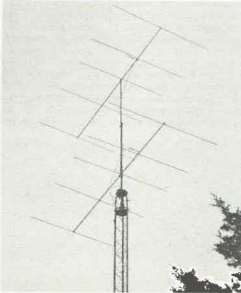
Fig. 9-16 — 5-over-5 stacked-Yagi array for 50 MHz, with all-coax feed.
