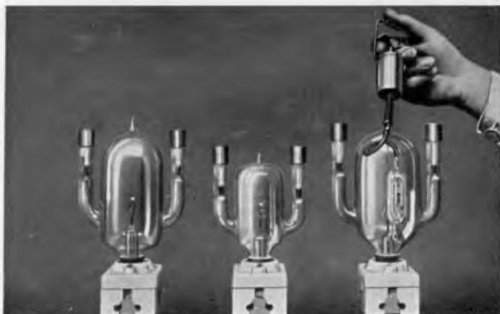
FIG. 86.—WEHNELT HIGH VOLTAGE VALVES.
