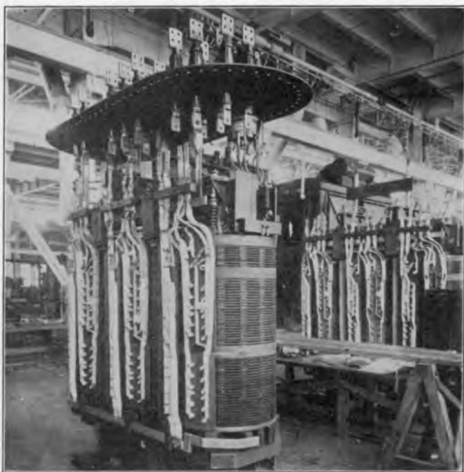
FIG. 83.—Brown Boveri transformer for 3,000-kw., 600-volt, 12-anode rectifier unit. The transformer is shown untanked.
