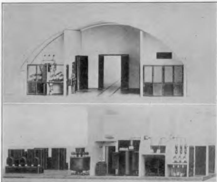
FIG. 191.—Model showing typical layout of Berlin elevated railway substation located under the arches of the elevated structure.
