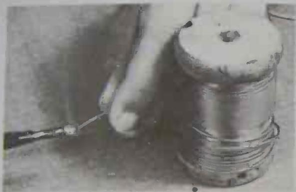
2. 'Tinning' the tip of the iron. When the iron is hot enough for use the solder will melt freely when touched on the tip.
