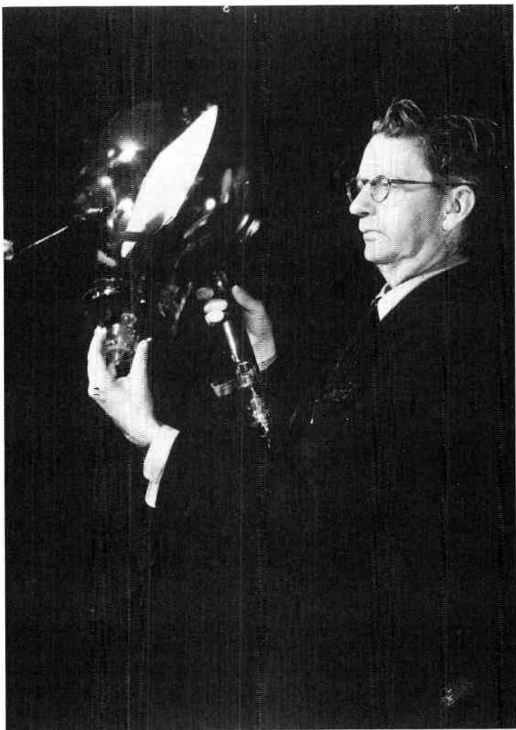
JLB with the Telechrome, the worlds first all-electronic colour tube from which all today's TV sets are descended.
