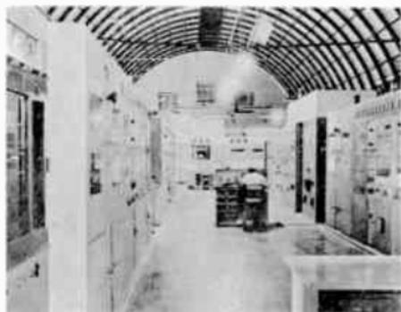
FEBC overseas transmitters located at Bocaue, Philippines. Equipment includes six 50,000-watt transmitters, one 10,000-watt transmitter and one 100,000-watt transmitter.
