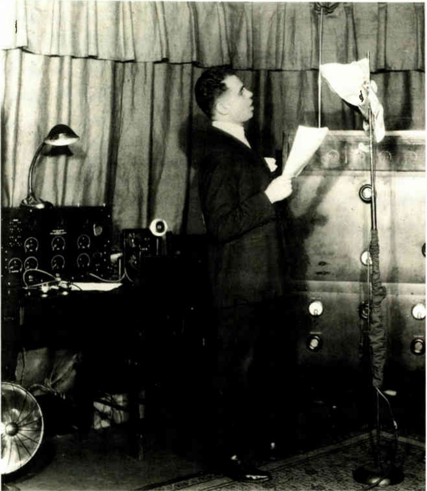
This photograph of an early broadcast studio (WDY in New Jersey) shows that acoustical design in 1921 included household drapes and a towel tied around the microphone for sound absorption. (Thomas C. Knight Collection, Series A, Box 3, Archives Center, National Museum of American History, Smithsonian Institution)
