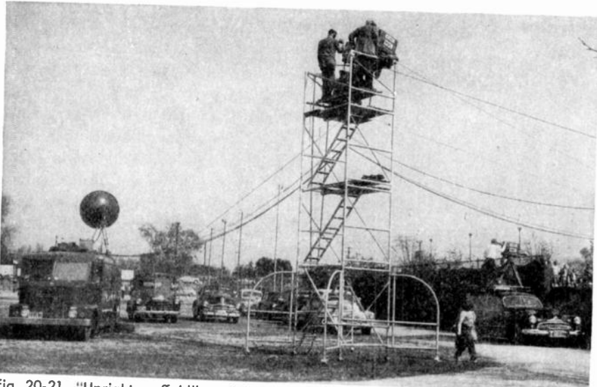
Fig. 20-21. "Upright scaffold" used for camera placements at Hollywood event (KNBH).
