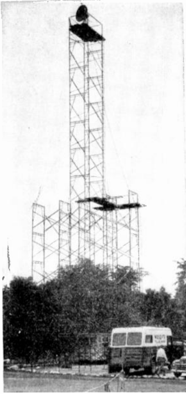
Fig. 20-22. Seventy-foot tower of scaffolding erected by WXYZ-TV, Detroit.
