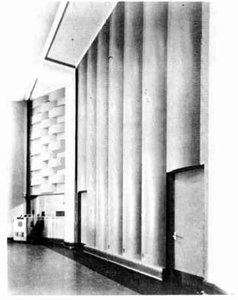
Figure 14-3 Vertical Poly-Cylinders. Note the control room window at the lower left of the picture.
