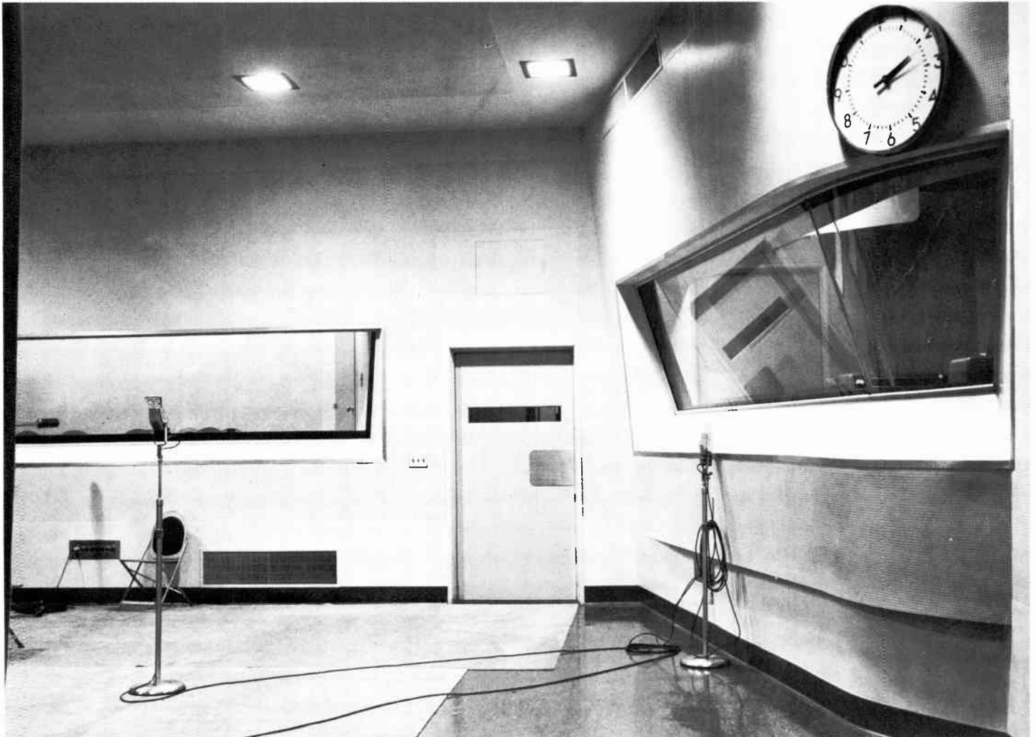
Figure 10-2 Studio-Control Room Window Courtesy Columbia Broadcasting System
