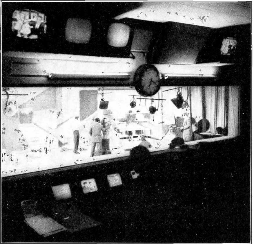
FIG. 83. Control room at a local station. WTVP, Decatur, Illinois.
