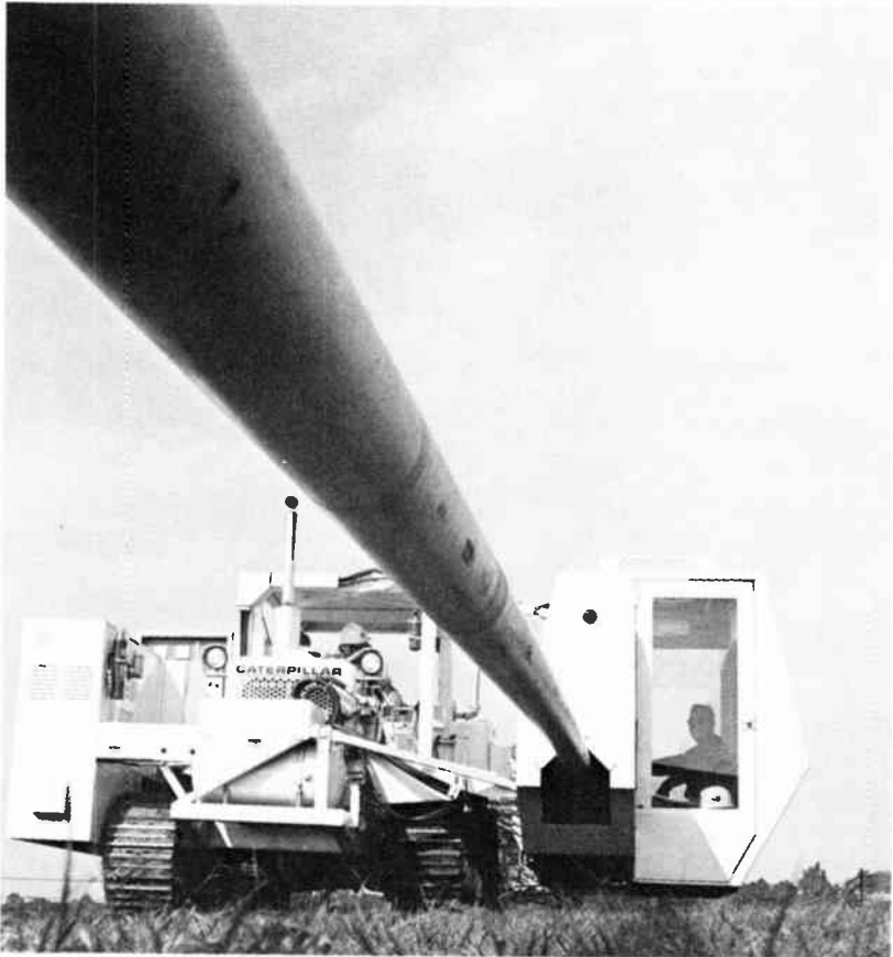
Figure 2-15 Section of circular waveguide being installed. Bell Labs Photo.
