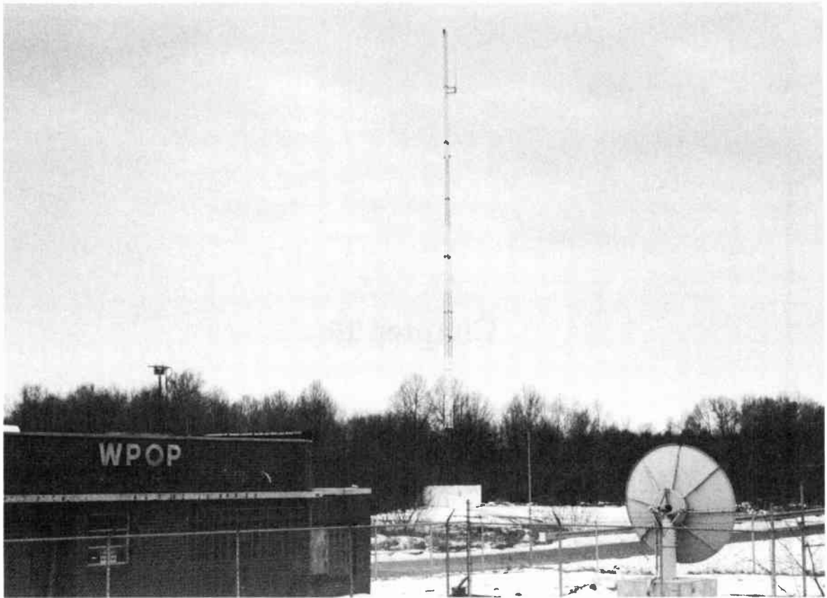
Fig. 15-1. Transmitter site. Many radio stations have studios in a central location, while the transmitter building and tower are out in the country. The satellite receiving dish (lower right) picks up network broadcasts that are relayed back to the studio. (WPOP-AM, Hartford, CT)
