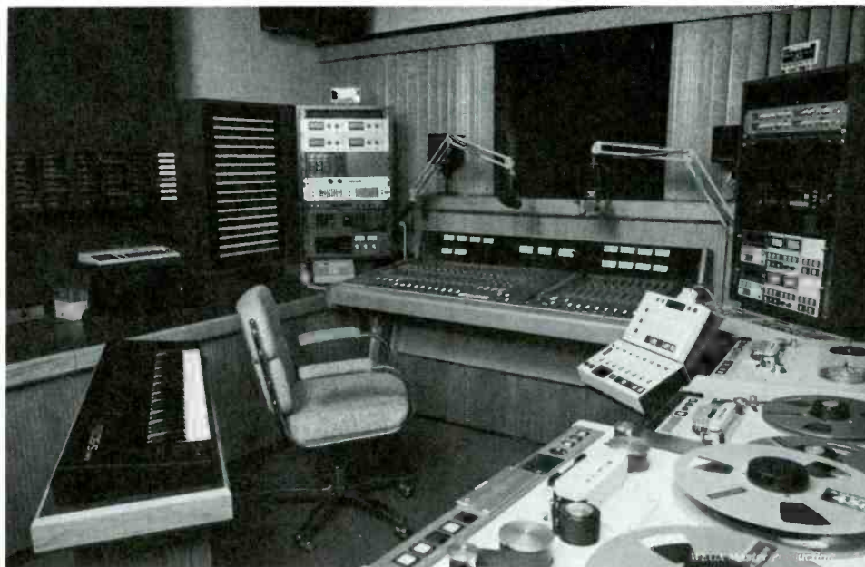
FIGURE 9.4 Although each production studio is unique, the basics of layout are fairly consistent from station to station. For the sake of ease and accessibility, most studios are developed in a U shape or a variation thereof. Courtesy WEGX and WHJJ/WHJY.
