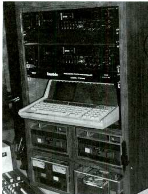
FIGURE 9.18 Equipment rack containing cassette tape machine, cartridge machines, and computer terminal. Rack mounted for convenience and ease of handling. Courtesy WMJX-FM.
