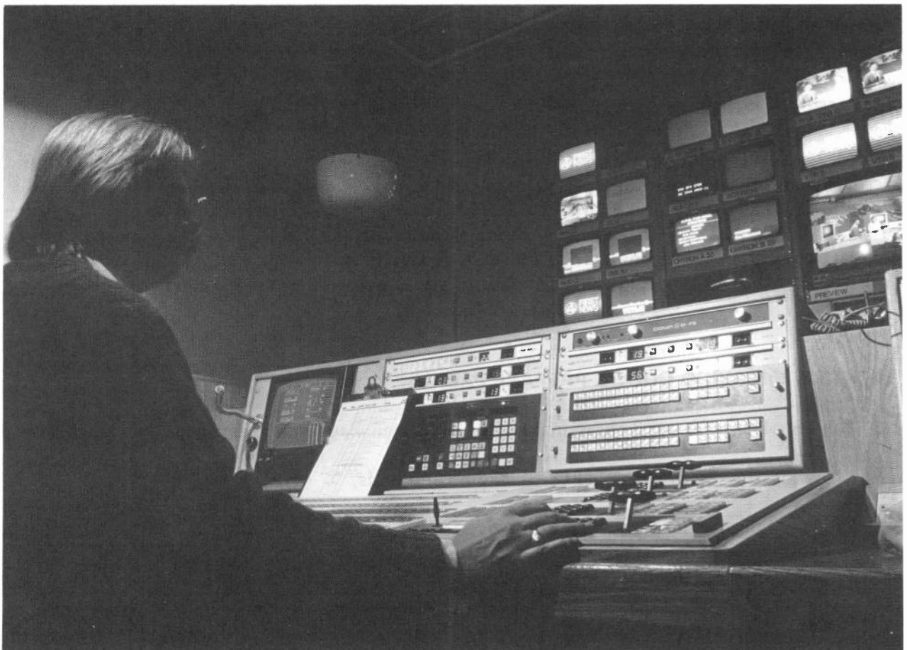
Figure 14-5. Entire live newscasts can be directed from this control room, or the facilities can be used for pre-production of complicated television news stories, complete with graphics and special effects.
