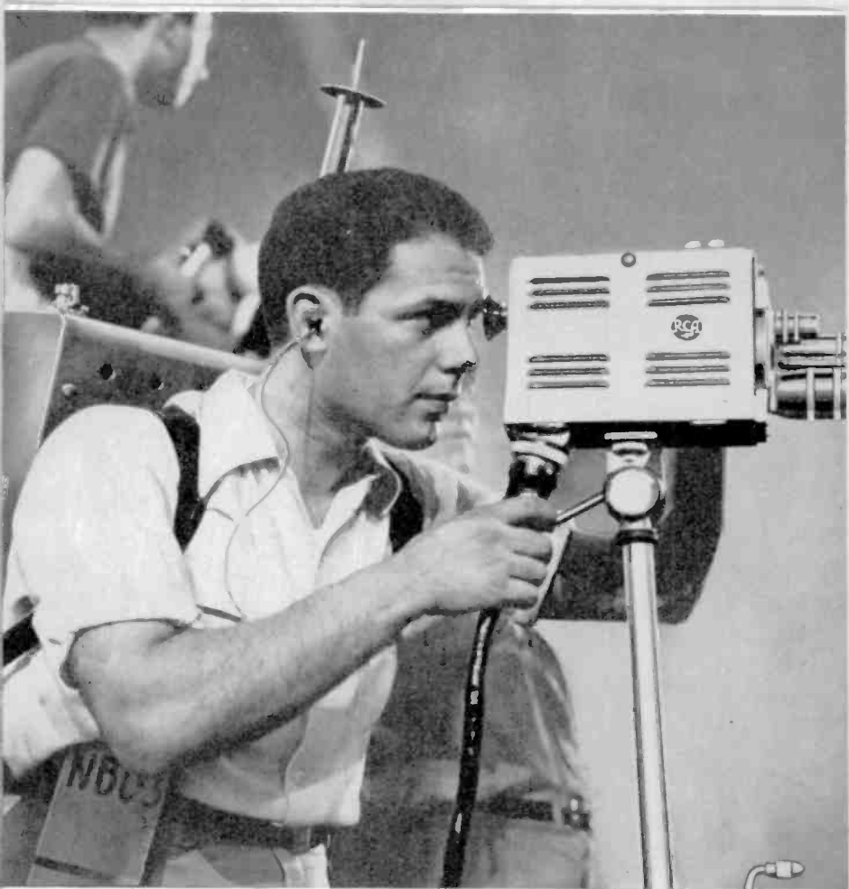
Here is the "walkie-lookie," a portable television camera and transmitter, used for the first time by NBC to cover the 1952 national political conventions in Chicago.
