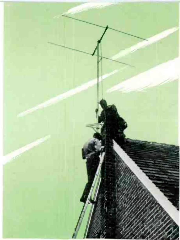
RCA servicemen erecting a television antenna.
