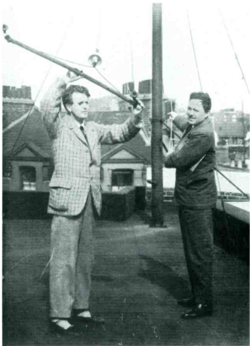
Erecting the Aerial at 2 T.V., the world's first Television Broadcasting Station.
