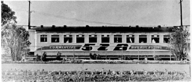
The radio station in a railway carriage — 5ZB.
