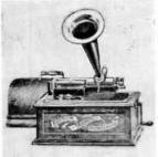
Edison "Triumph" phonograph of 1898 could play fourteen two-minute records per winding of its triple-spring motor. It was supplied with a 14-inch brass bell horn and sold for \$50.00. (O. Read collection.)
