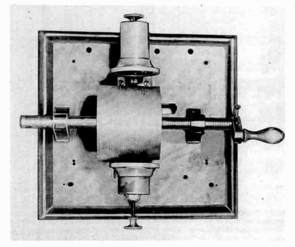
Fig. 2-4. Constructional details of Edison's tinfoil phonograph are shown including both "speaker" and "reproducer." (Courtesy of Edison National Historic Site.)
