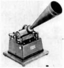
Edison "Gem" phonograph, 1901, with improved spring motor and start-stop-regulating device. A gear-change attachment (added later) reduced rotation speed of feed screw so that four-minute records could be played. (O. Read collection.)
