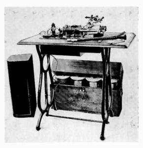
Edison battery-operated "Spectacle" phonograph of 1889 was mounted on a sewing machine stand. Box contained four wet cells (Edison-Lalande) to supply about five amperes current to the DC motor. (Edison National Historic Site Museum.)
