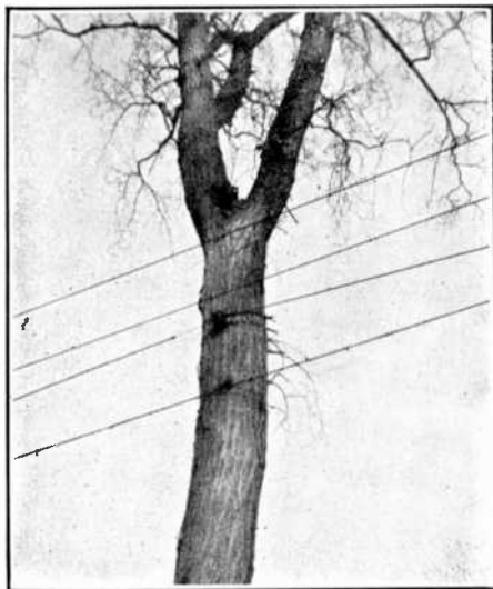
FIG. 91. Tree grounds are an easily avoidable source of interference.
