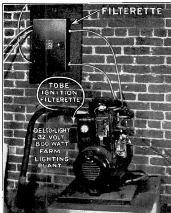
FIG. 76. Typical installation of Filterette DM-32.
