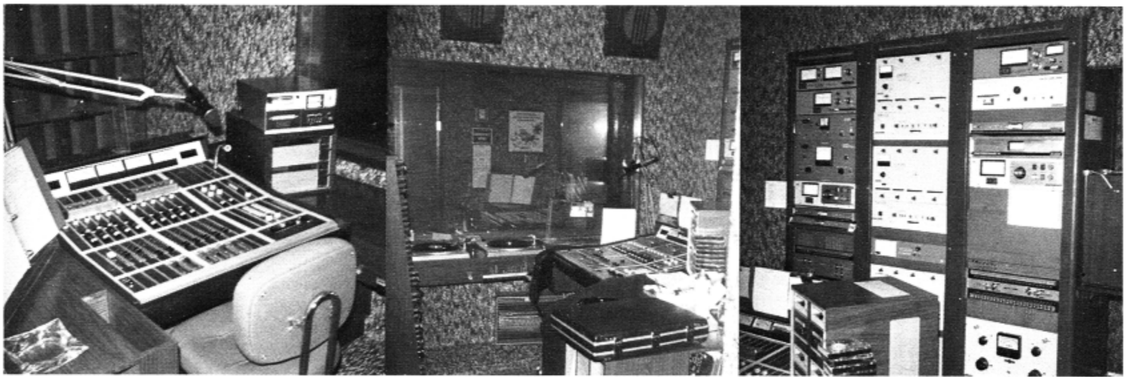
On-air control room at CKOT, like adjacent master control (centre), is equipped with McCurdy SS8500 stereo console. Photo at right shows main monitors in master control: FM, STL and AM (left to right).
