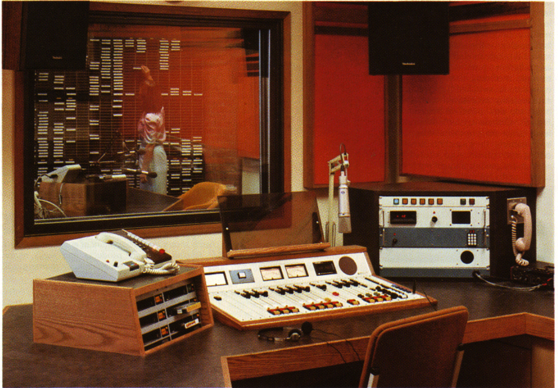
Photo 7: C-FAX news booth. The announcer in this room has a good view of the main control room and adjacent sports booths. Since all music is on cartridge, this room has all the facilities required for an emergency on-air studio. The auxiliary equipment turret on the right contains remote control room switcher, digital thermometer, mobile intercom facilities and remote access to the crossbar facilities. Judi Vertes Helfrich, traffic director, is in control room.
