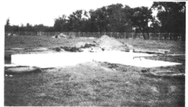
Photo 3: Abandoned pipes and structures were part of filtration plant.
