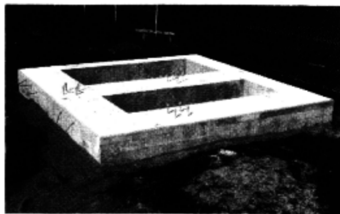
Photo 5: Finished foundation for one of towers is supported by filter bed roof.
