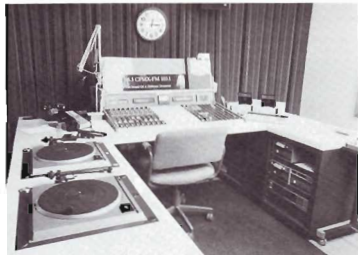
The Cobourg master control room of CFMX-FM includes a McCurdy board, two technics turntables, a pair of Phillips CD players and Revox reel-to-reel units.
