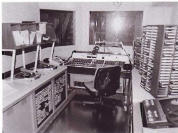
Master Control Room at CFDA Victoriaville with its McCurdy Console.
