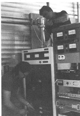
Cliff Wheeler (bottom) and Kelly Klassen install new transmitter.
