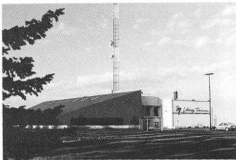
And after expansion and renovation.
