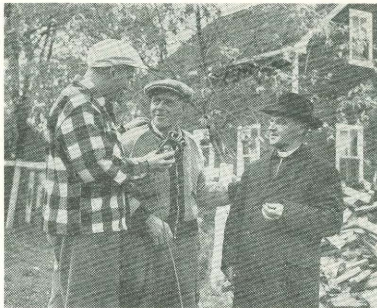
Recently, because of power developments on the Winnipeg River, it became necessary to move a considerable part of the village of St. George, Manitoba, from its original site, as flooding caused by the power dam would have inundated it. CBC's Saturday Magazine (Saturdays, W-2:03, K, X-1:03 p.m.), covered the event. NORMAN McBAIN, CBC announcer (left), here interviews DIDAS WILCOTT, local farmer whose home had to be moved, and FATHER J. A. D. McDUGALL, parish priest of St. George.
