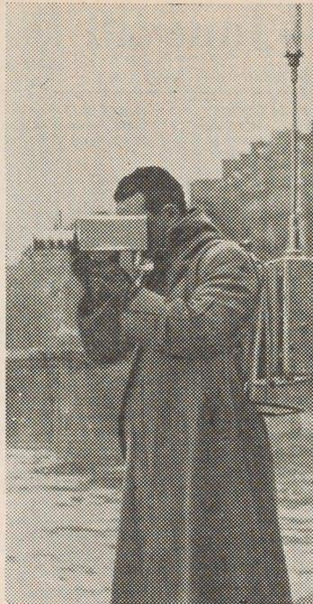
**PORTABLE TV CAMERA** developed in France is used by CBC to cover parts of the Royal Tour. The battery-operated transmitter is carried on the operator's back.
