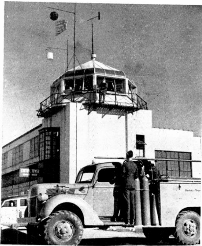
The Control Tower, the nerve centre of every airport.
