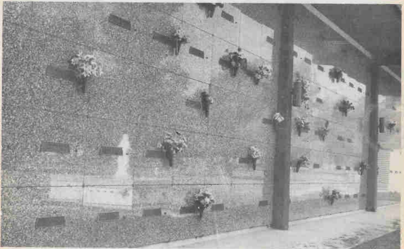
Fig. 8. Typical crypt structure with granite closure plates is shown — a temporary time capsule repository. Presence of capsule can be confirmed periodically with beat-frequency metal detector. See text.
