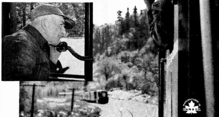
The Algoma Central Railway credits 2-way radio with saving considerable time on every round trip with long freight trains. Fixed and portable sets in locomotive and caboose allow the crews to keep in constant contact with the engineer. The conductor and engineer can check orders instantly, speed instructions and consult in respect of work to be done.
