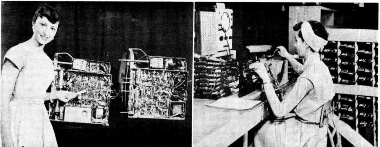
● *Left:* A new method of assembling television sets using "printed wiring" results in the much simpler assembly of the chassis at left as compared with the old type. *Right:* Testing of the many individual components constituting a complete printed wiring circuit is simplified with this special comparator.
