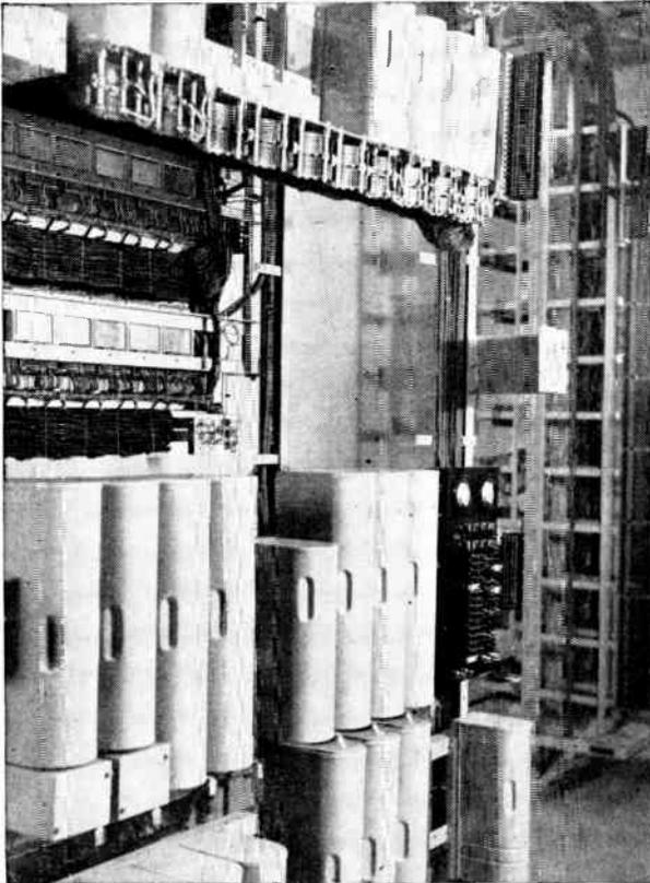
*View of the compact, efficient STROWGER Automatic installation at Newcastle. A similar unit will be installed at Welcome.*
