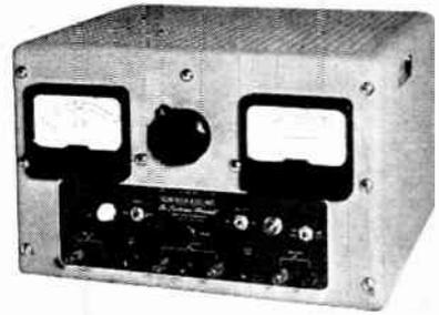
We have been repeatedly advised of the need for a laboratory power supply with current capacity of up to one-half ampere. During the design of the unit it appeared desirable that it should embody characteristics making it suitable for pulse work.
