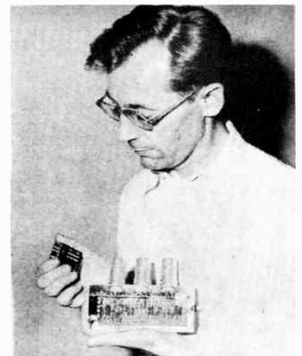
● Comparison of transistor and conventional tube circuit.
