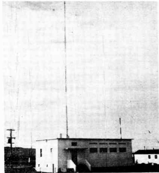
● Fifty foot antenna tower carrying three special type antennas supplied by Rogers Majestic Electronics Limited.
