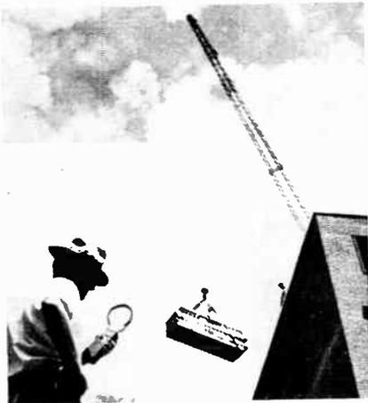
The Handie-Micro-Talkie transmitter may be used with any standard F.M. mobile set or base station operating on the same frequency. Subminiature dry battery power supply uses standard 30 and 1.5 volt cells, providing up to 30,000 ten second transmissions on a set of "B" batteries; up to 15,000 ten second transmissions on a set of "A" batteries. There is no stand-by current drain, power is consumed only while transmitting.
