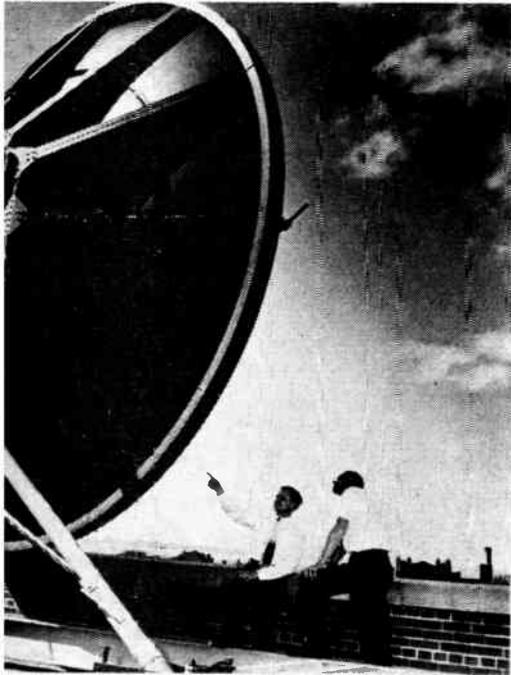
● Canadian Westinghouse electronics engineers who worked on year-long project to develop new communications system check positioning of transmitting antenna. It is aimed at Kinmount, Ont., 130 miles away from Hamilton. Tests were carried out between Hamilton and Kinmount.
