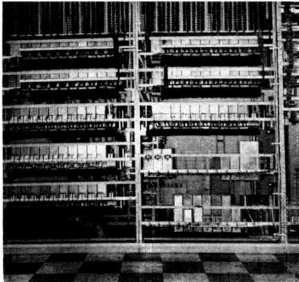
*Above: View showing close-up of the private exchange (PAX) installation. Right: An overall view of the exchange installation.*
